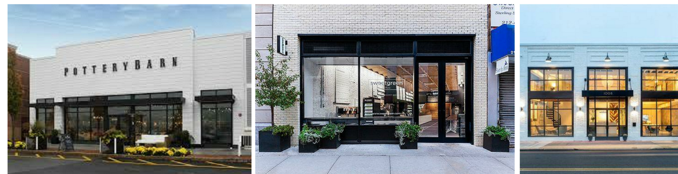
THE WHITE BRICK BASE - STOREFRONT
